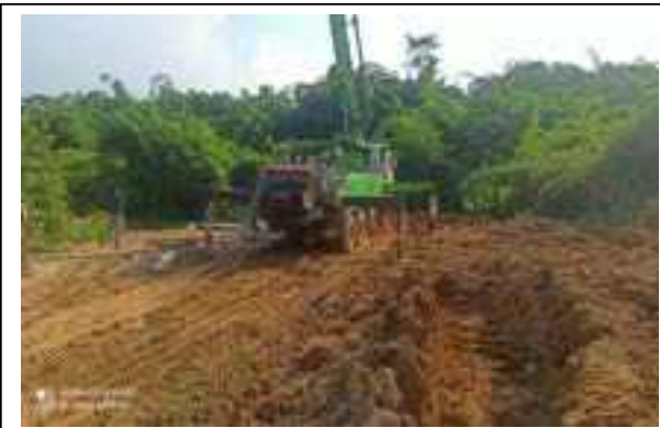
Undergoing construction of the approach road
