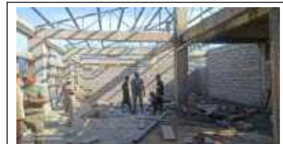
Undergoing construction sites in indoor sports complex
