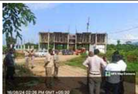
Construction site of Assistant Commandant Block
