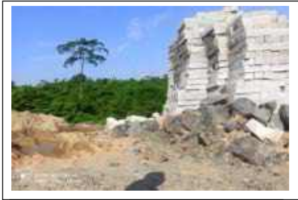
Brick block material inside the proposed site
