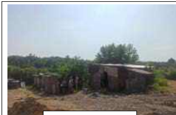
Temporary Labour shed
