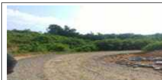
Constructed road inside the proposed area
