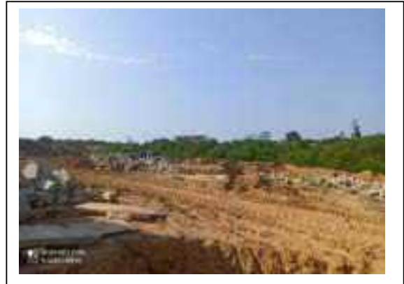
Levelled Parade Ground site
