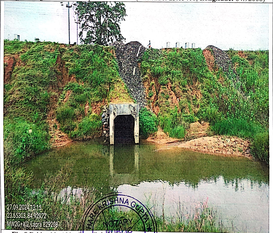
Fig:8 Bridge No 132 - Box Culvert Type (Latitude: 23.65303, Longitude: 84.92972)
