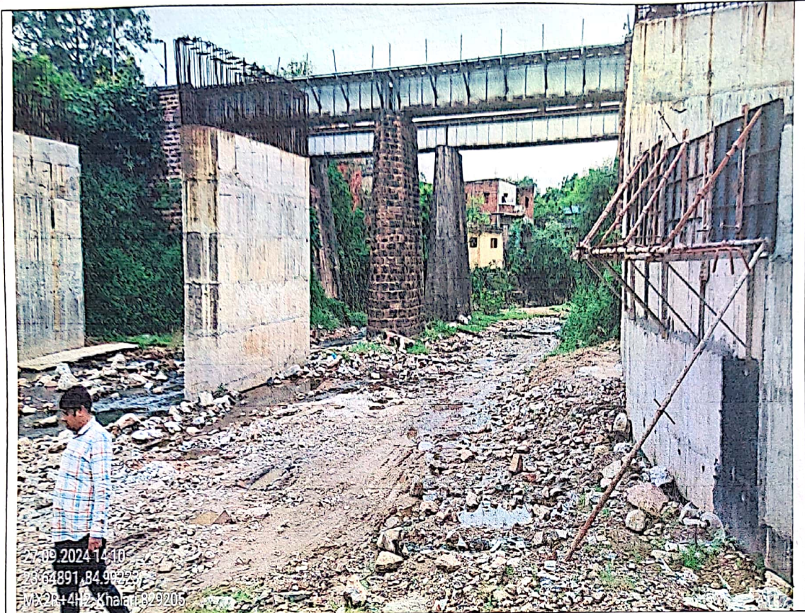
Fig:11 Bridge No 120 at Khalari Bazar Tand (Latitude: 23.64891, Longitude: 84.99223)
