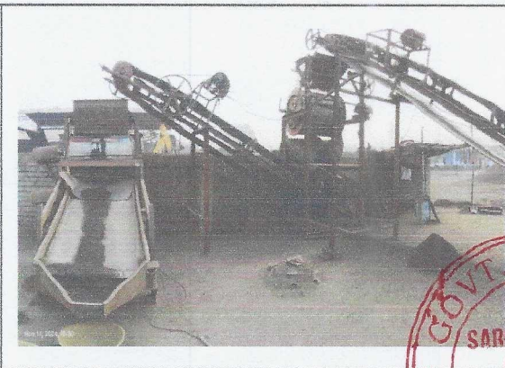
Pic. 6: Operation of Screen unit - 1 at Al Kia
