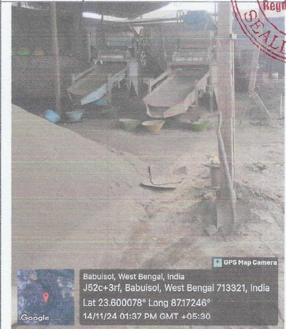
Pic. 8: Magnetic-separator & Fixed-screen-3
