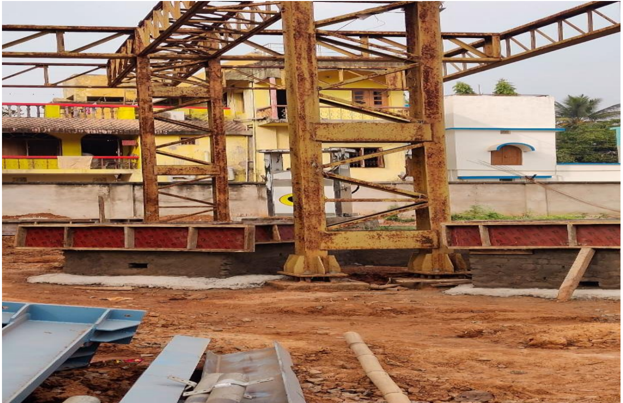
PHOTOGRAPH DATED 26/11/2024 SHOWING LARGE SCALE CONSTRUCTION OF CNG STATION
