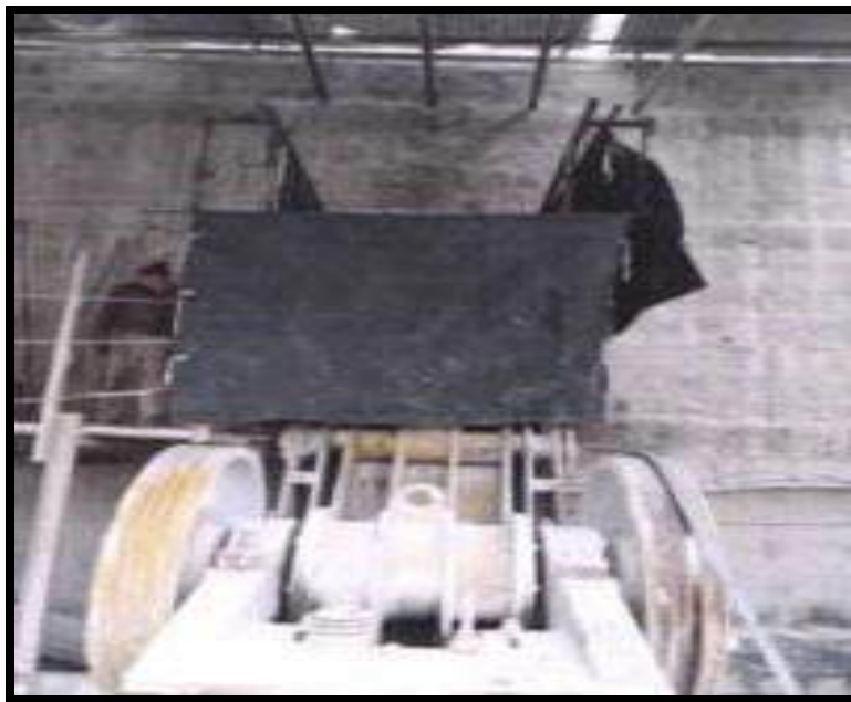
Figure-1: Covering of Primary/Jaw crusher
