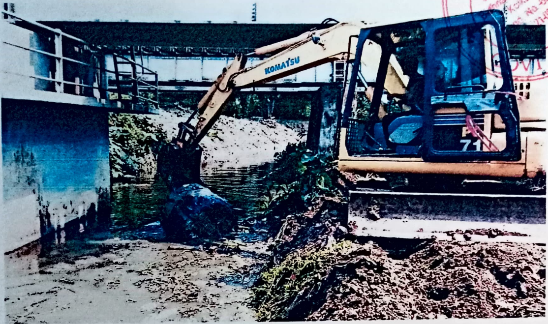
Work Below Howrah – Kharagpur S.E.Rail Line , Masila Sankrail
