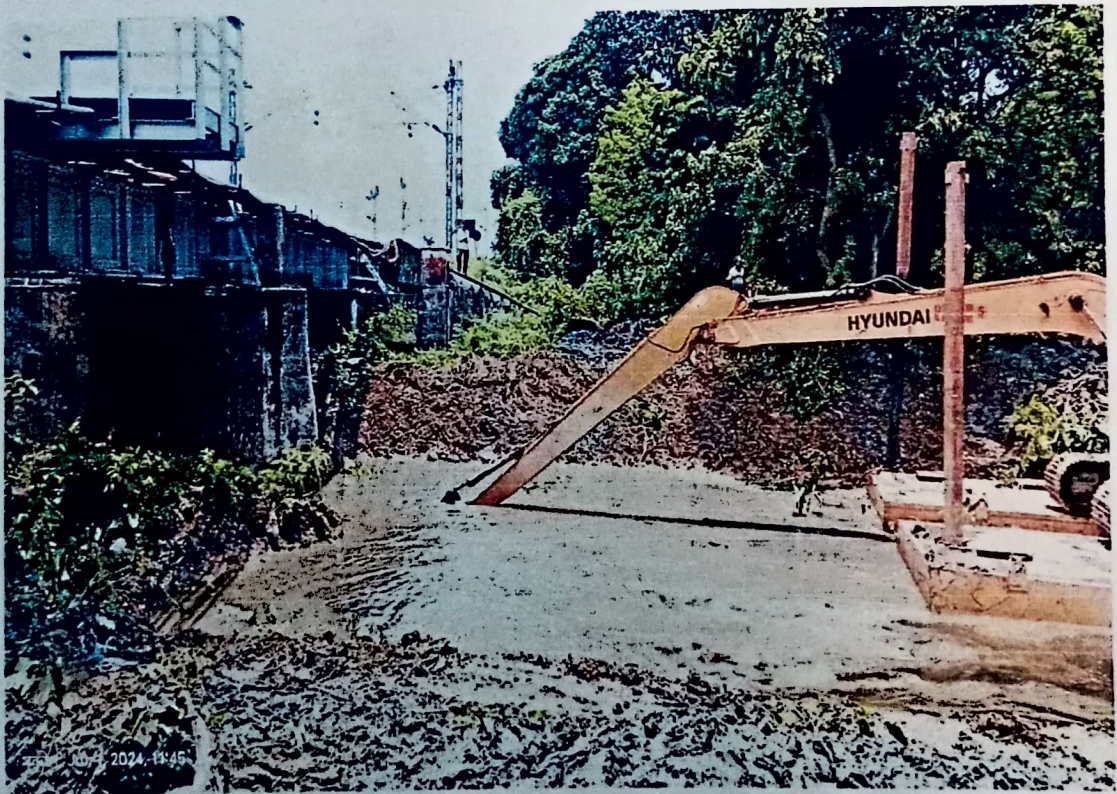
Work Upstream of Howrah – Kharagpur S.E.Rail Line , Masila Sankrail
