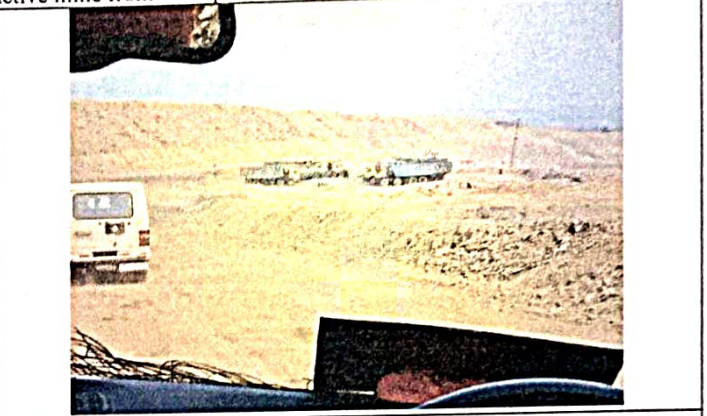
Pay loaders stationed at the site
