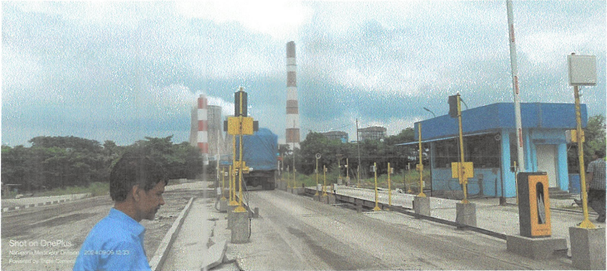
Figure 1 – A bird's eye view from the Weigh bridge side
