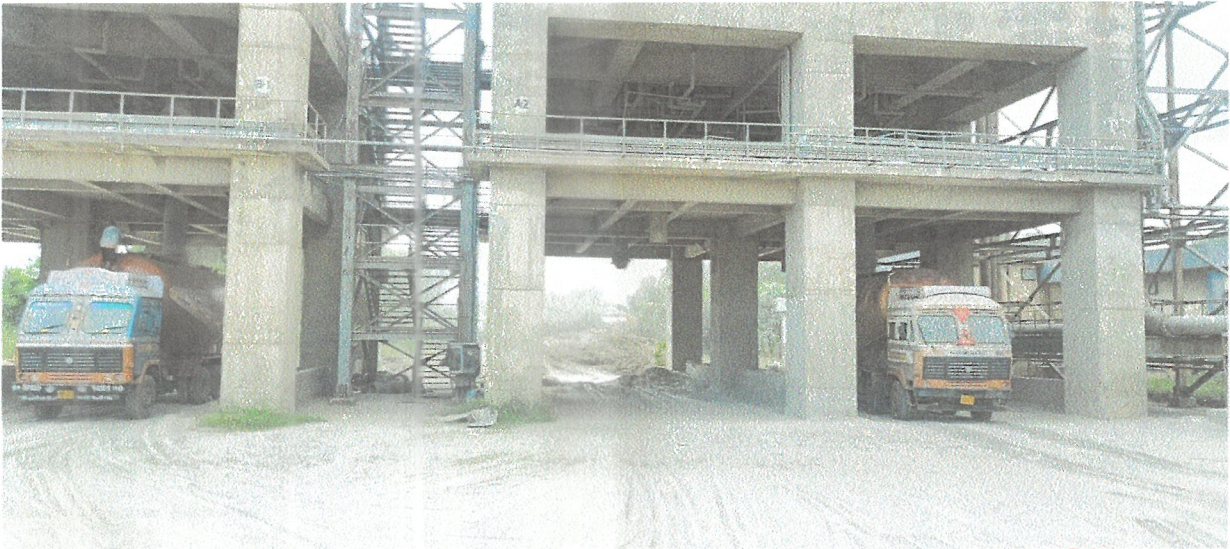
Figure 2- Filling of the bulker from fly ash silo
