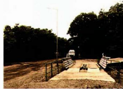
Fig 6: Mechanical Wheel Washing System near Raw Material Gate
