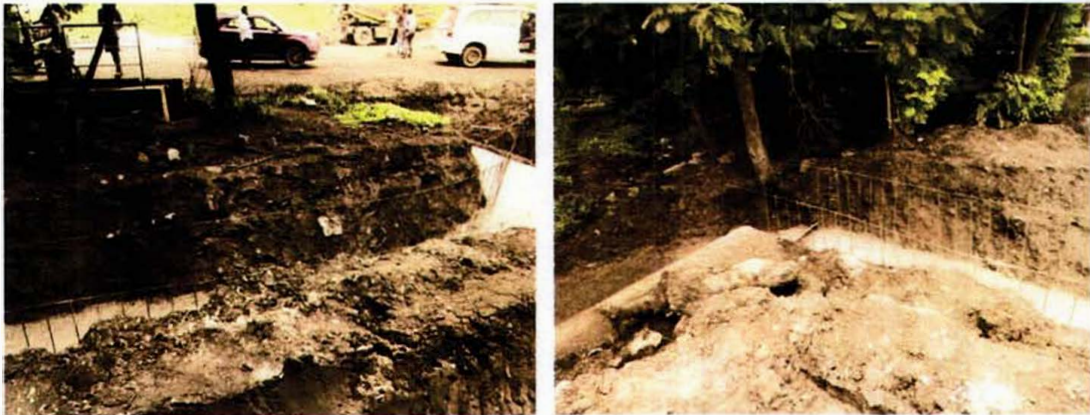
Fig: 8 Road side drain constructed by IDCO at the JCDL Road
