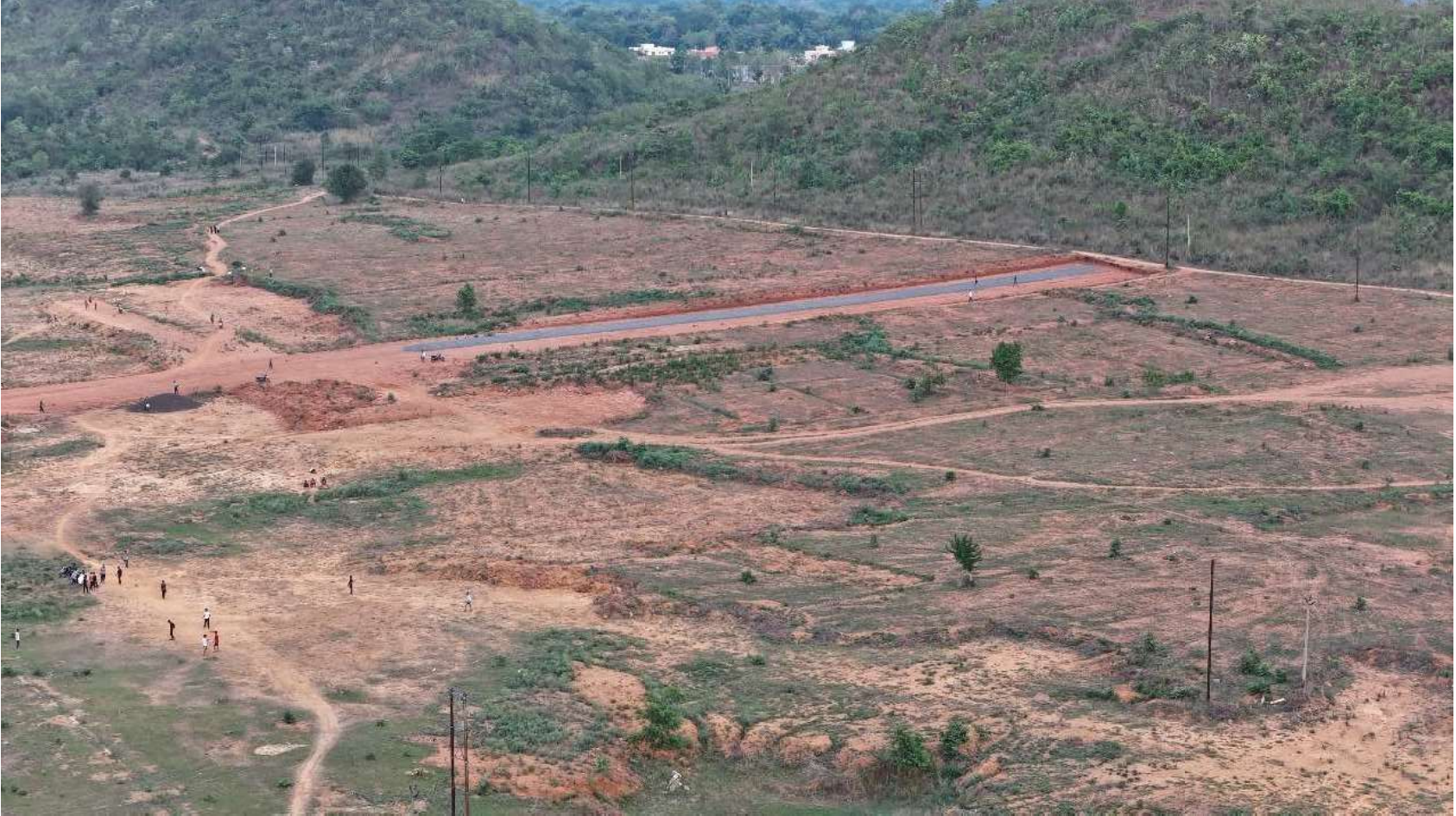
Photograph showing constructed metalled road in PF 450
