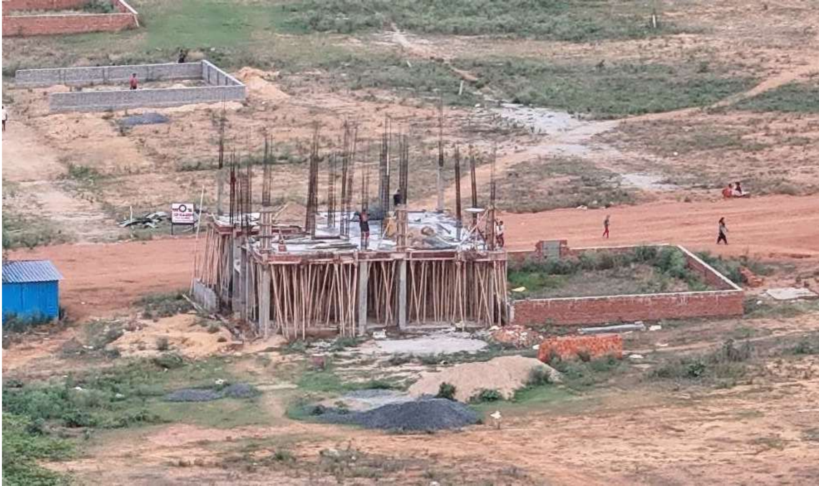
Photograph showing ongoing construction in PF 450
