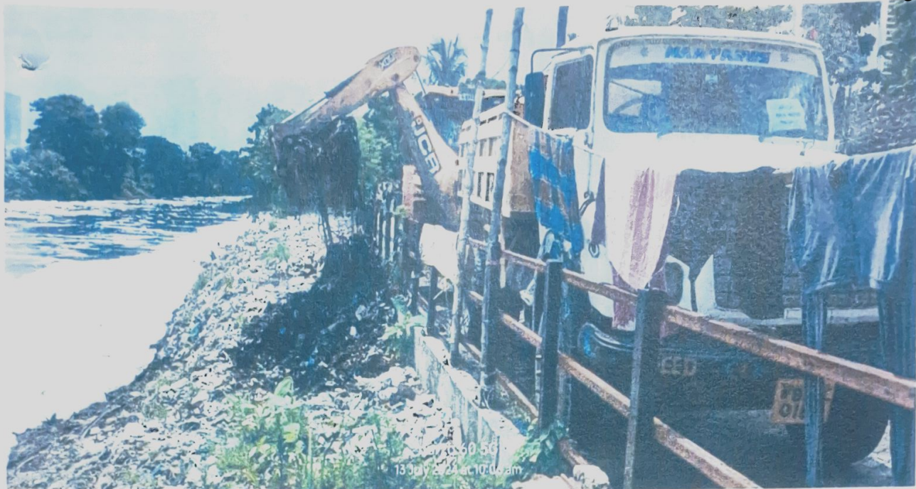
WORK ONGOING PICS
