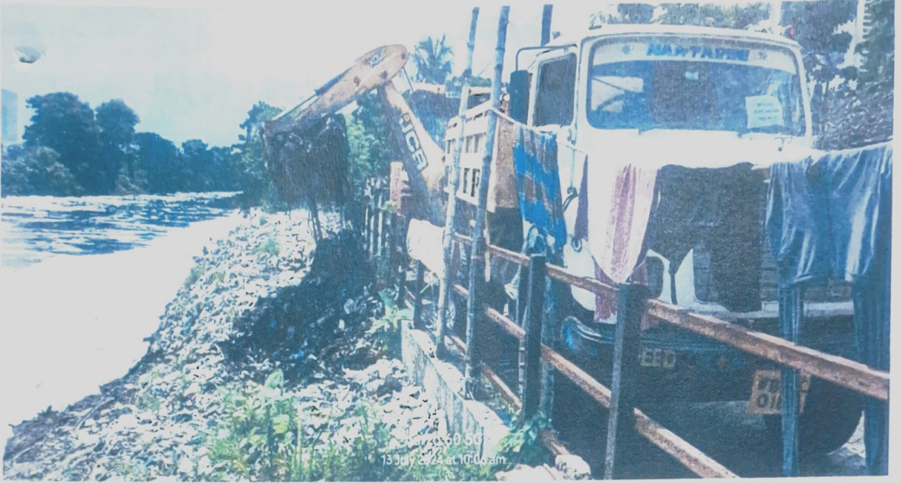
WORK ONGOING PICS
