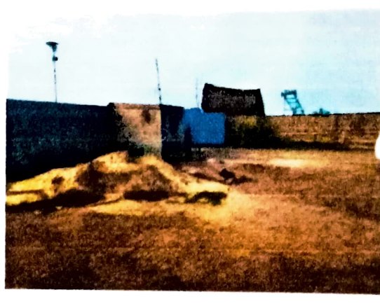
Pic. 12: No plantation/green-belt along boundary walls
