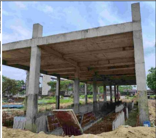
Photo 4: Another view of new construction activity near sinter plant area
