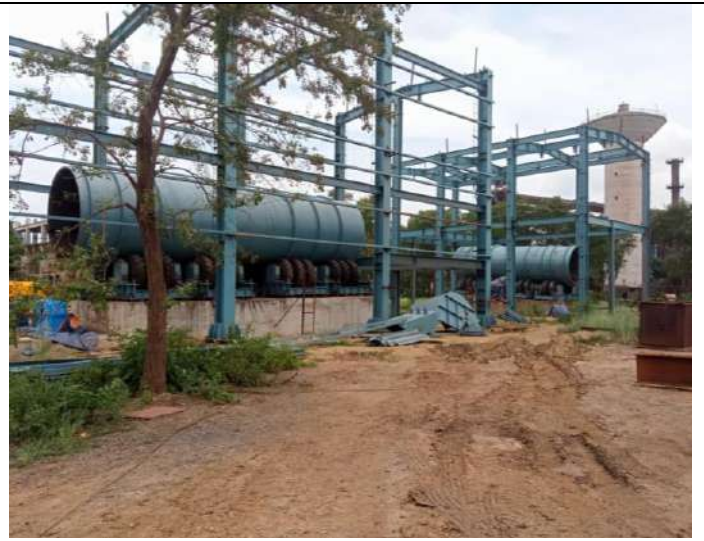
New incomplete construction activity
