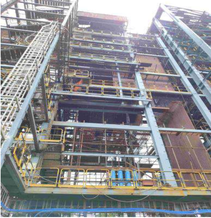
Repair activity in DRI
