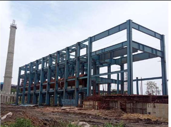
New incomplete construction activity
