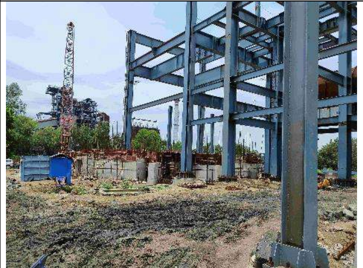
New incomplete construction activity
