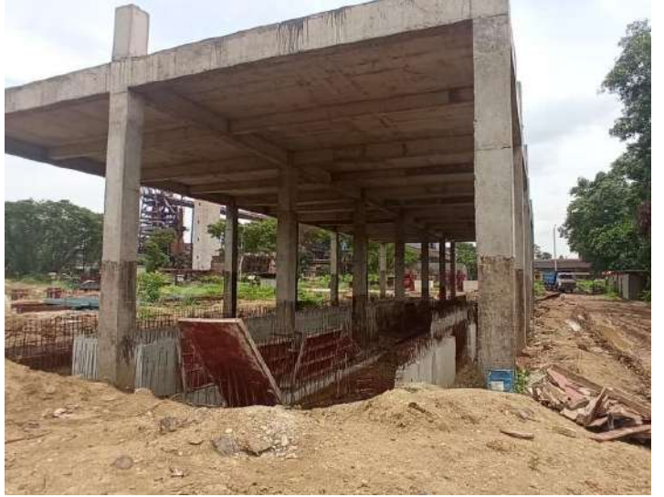
New incomplete construction activity
