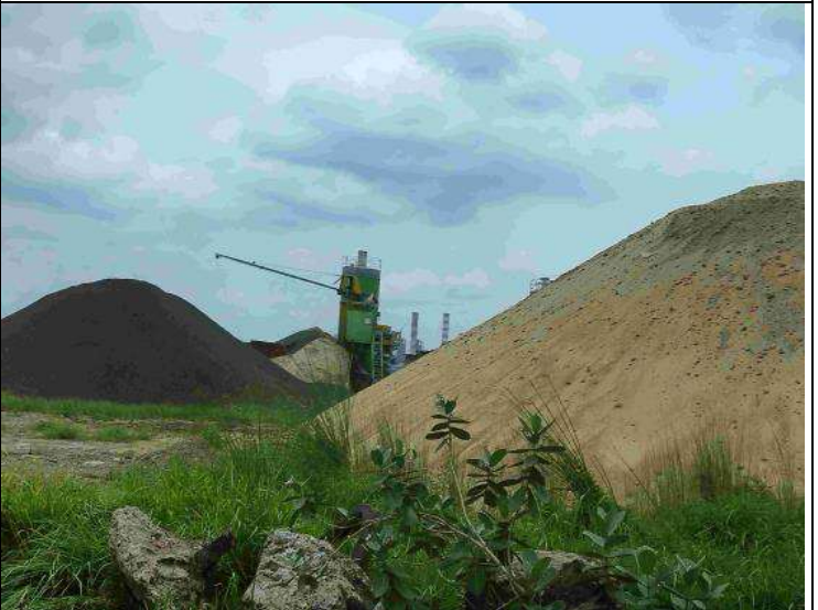
View of batching plant
