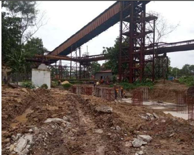
New construction activity near blast furnace
