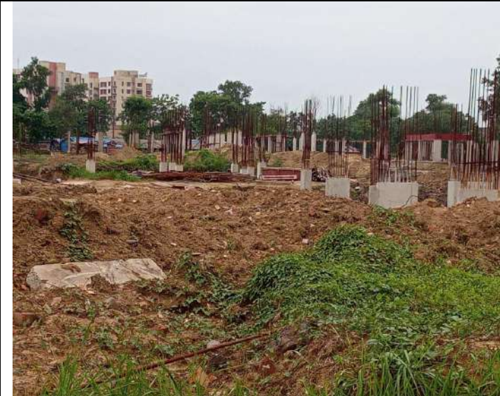
New incomplete construction activity
