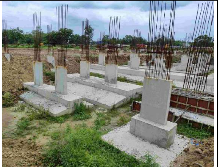
New incomplete construction activity
