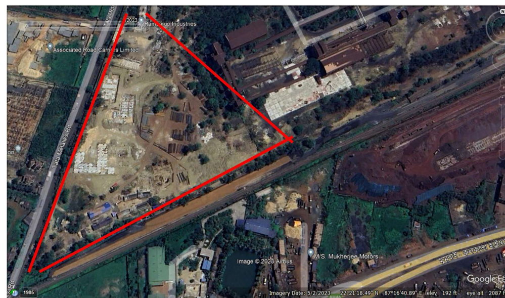
Part of the Proposed Pellet Plant Area in dated 02.05.2023
