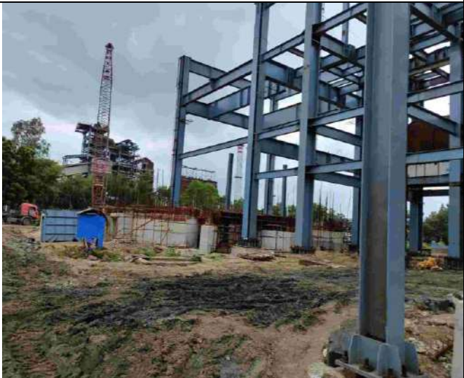
Photo 3: New construction activity at the proposed sinter plant area
