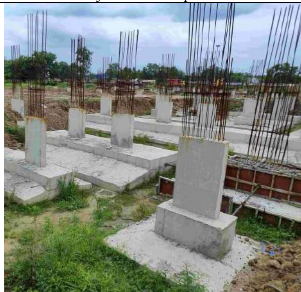
Photo 6: New construction activity near the present office building
