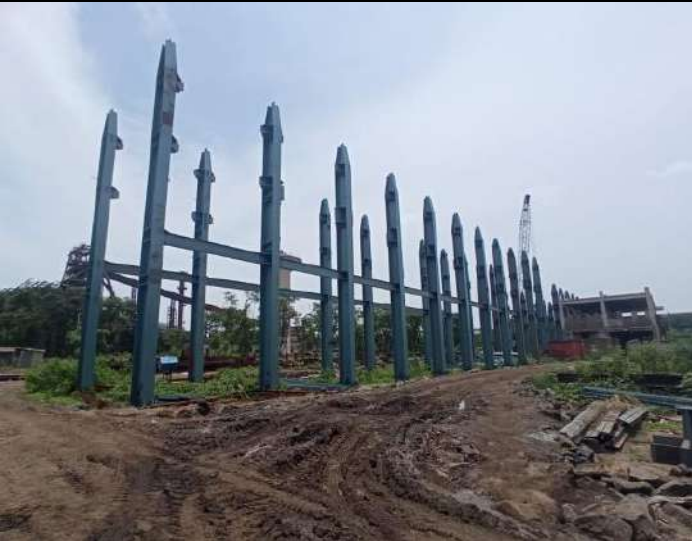
New incomplete construction activity
