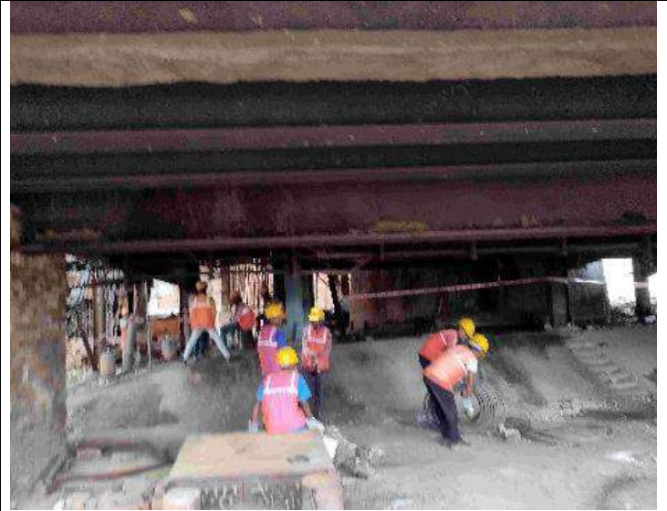
Repair activity in Blast furnace
