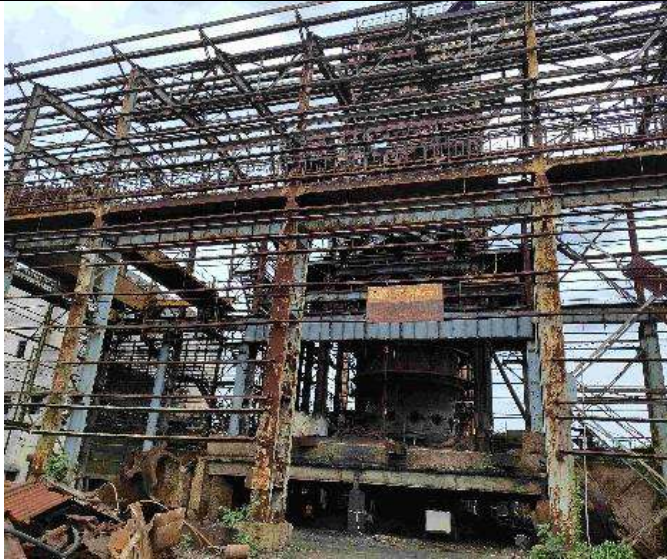
Repair activity in Blast furnace
