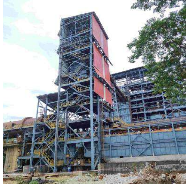
Repair activity in DRI
