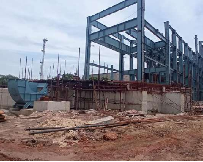
New incomplete construction activity
