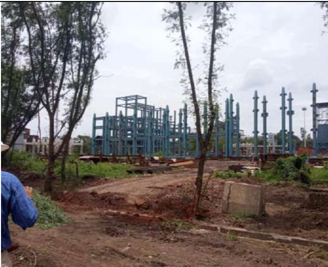
New incomplete construction activity
