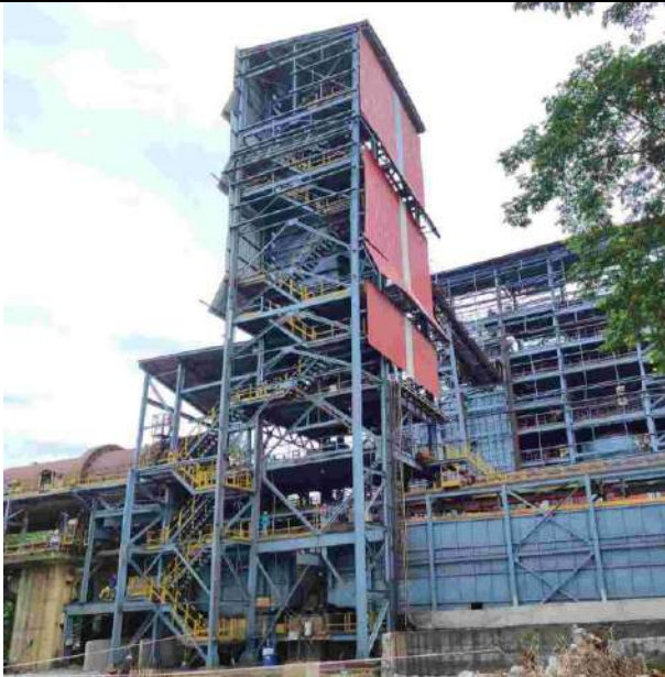
Photo 1 : View of repairing activity at DRI unit
