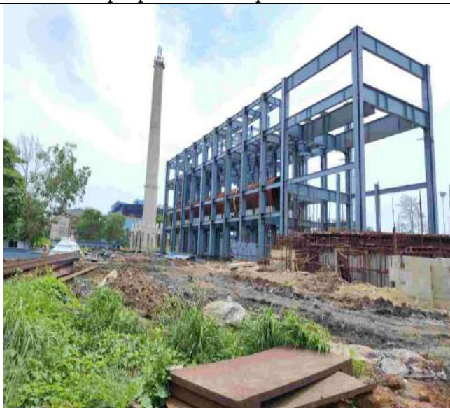
Photo 5 : Incomplete new structure at the proposed sinter plant area
