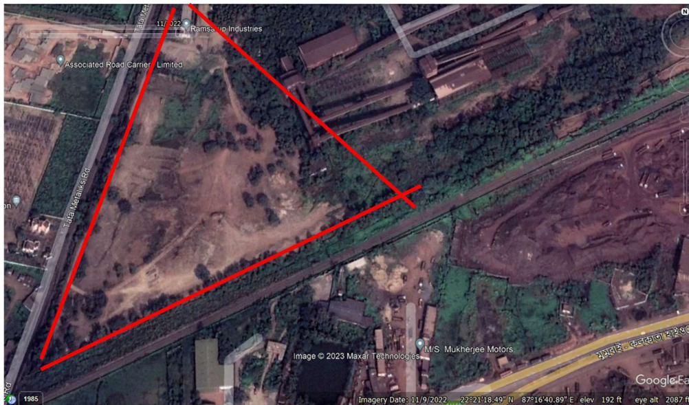
Part of the Proposed Pellet Plant Area in dated 09.11.2022
