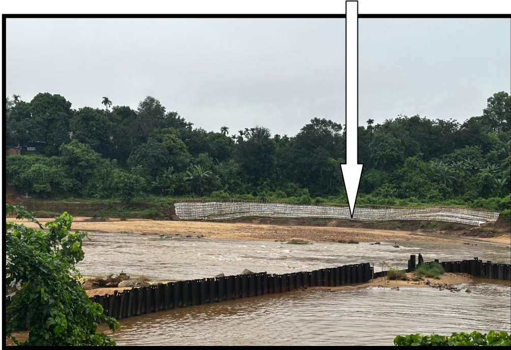
PARASIDING AND SAND FILLED BAG WITH BAMBOO SUPPORT – LEFT SIDE
