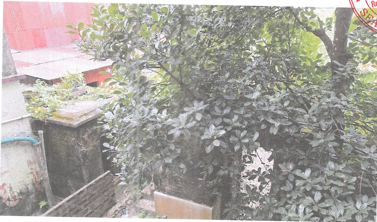
View of the tin roofed unit from the complainants residence
