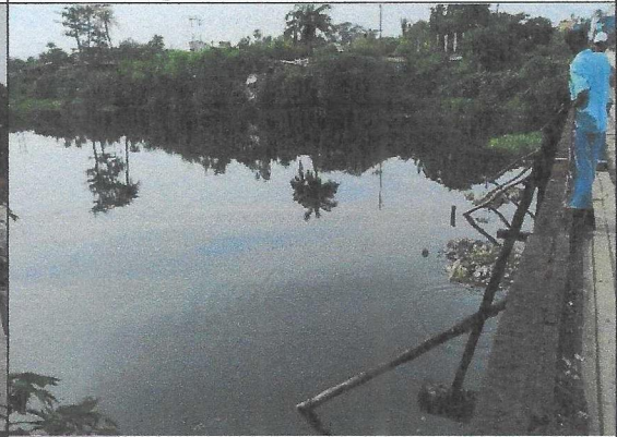
Fig.15: SWF (Basanti Canal) at Downstream
