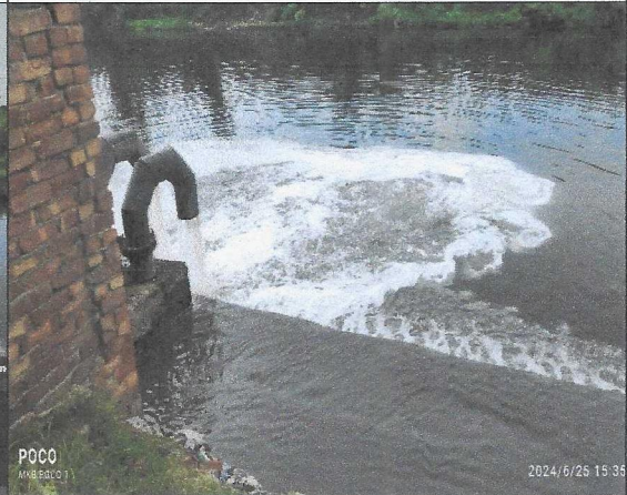
Fig. 13: Canal 3 at Gate No.3
