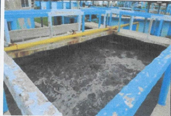
Fig. 5: Sulphide Tank
