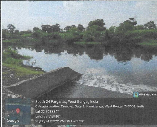
Fig. 12: Canal 2 at Gate No.2
