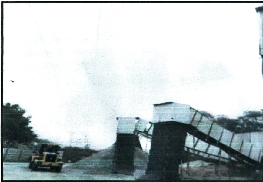
Figure-2(a): Chute from top of discharge point
