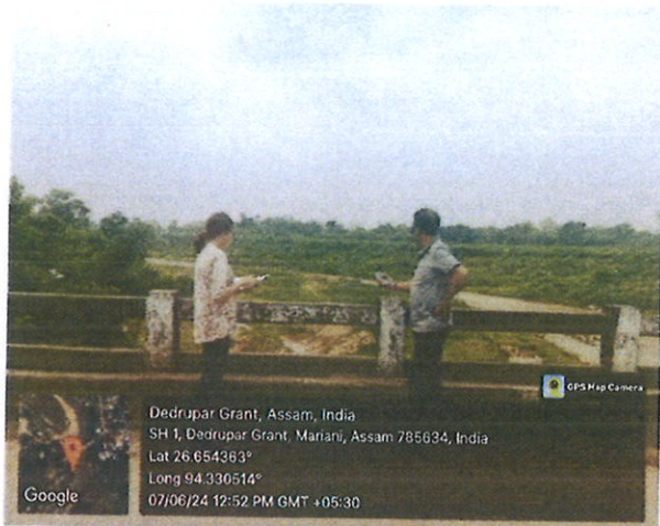
Sand excavation site at Mariani Bhogdoi Bridge
