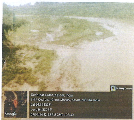
Sand excavation site at Mariani Bhogdoi Bridge
