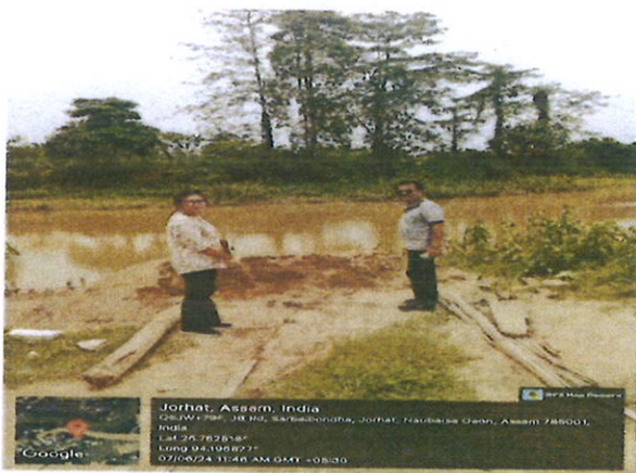
Sand excavation site near Rajotiya Sarbai Bandha gaon, Jorhat
