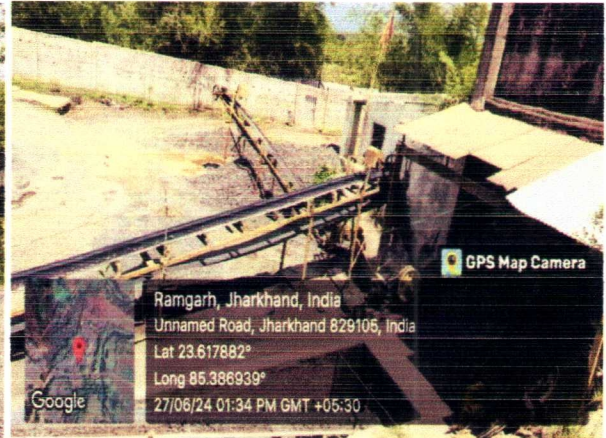
Photo 46: Photo of water spraying arrangements
