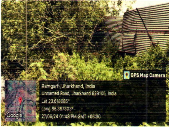
Photo 57: Photo of metal sheets with pucca boundary wall.
