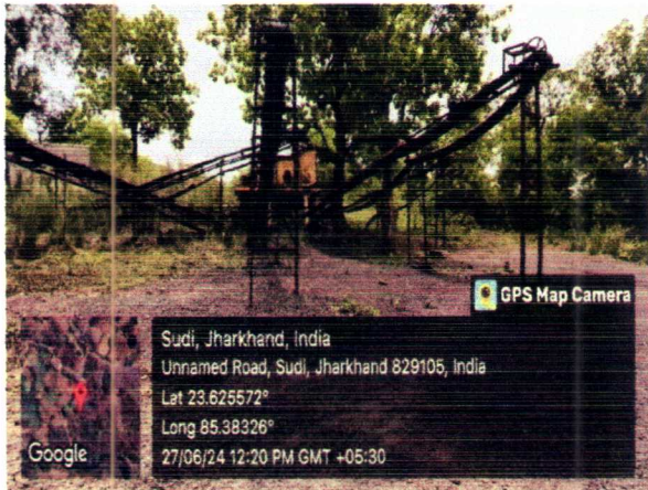
Photo 13: Photo of inoperative crusher unit.
