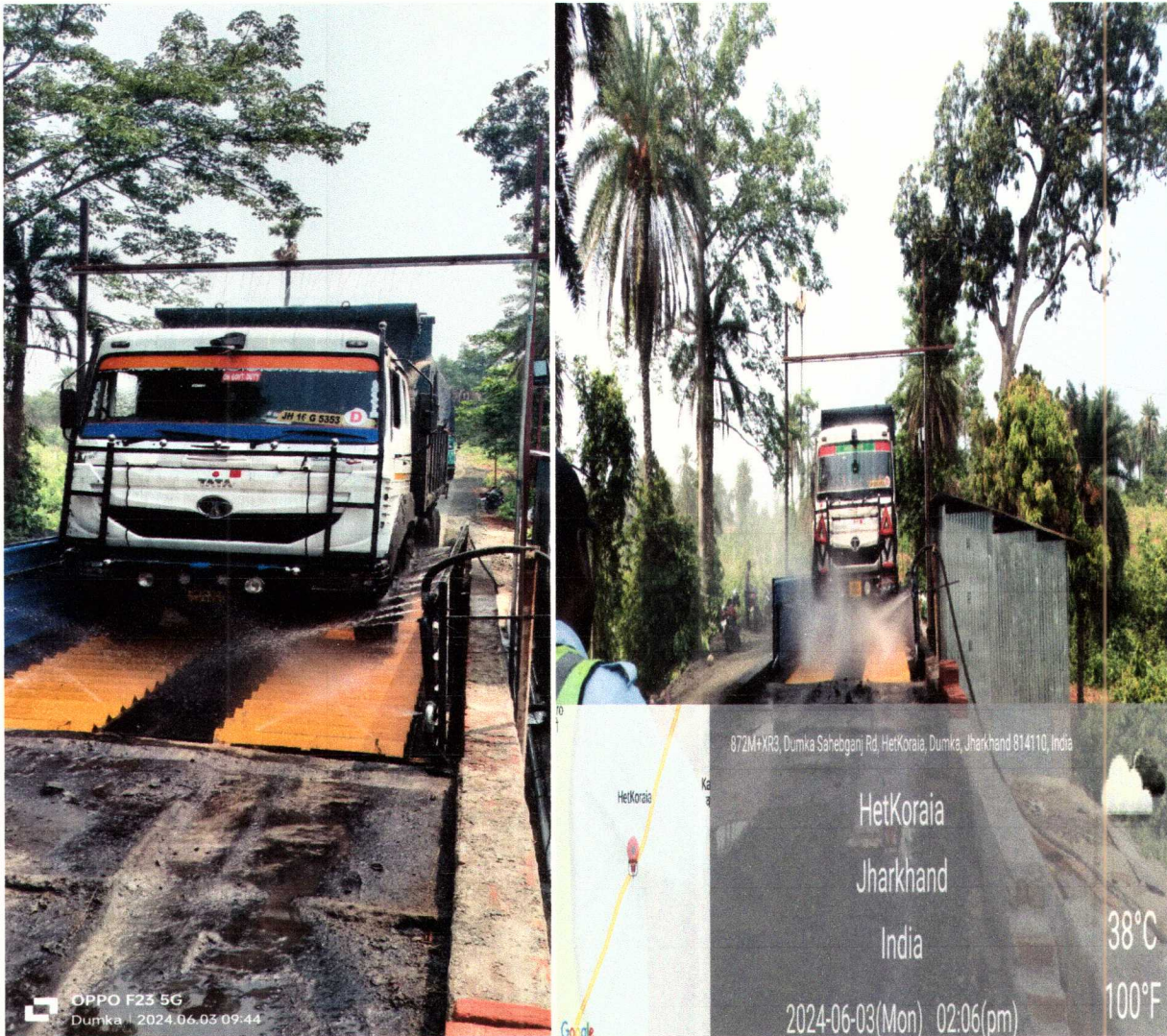
➤ Wheel Washing facility at Hetkoraia.
