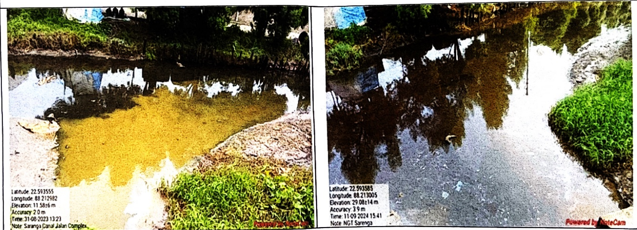
Pic. of drain from Jalan Industrial Complex
