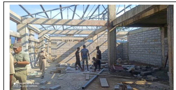
Undergoing construction sites in indoor sports s complex
