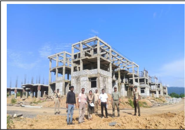
Construction site of Commandant Office Block
