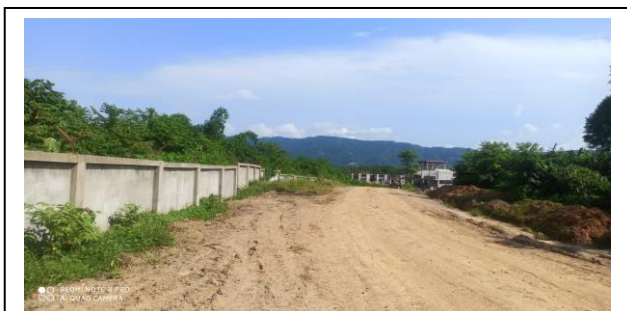
Constructed Boundary wall of the proposed site
