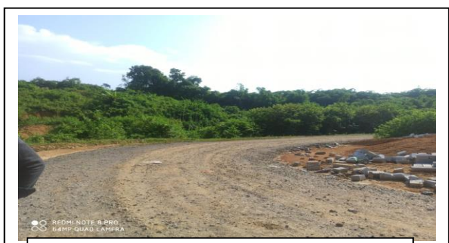
Constructed road inside the proposed area
