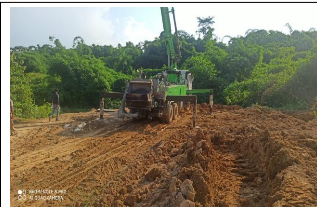
Undergoing construction of the approach road
