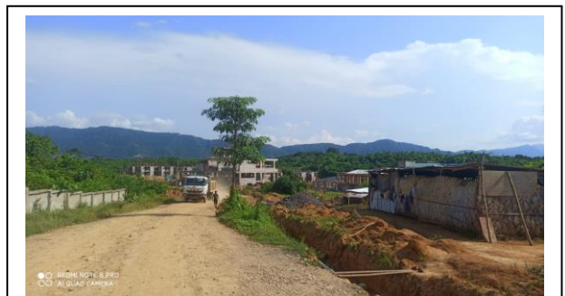
Boundary wall and proposed site
