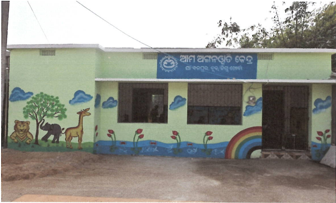
Repairing and water supply of Balapur AWC (Work on progress)
