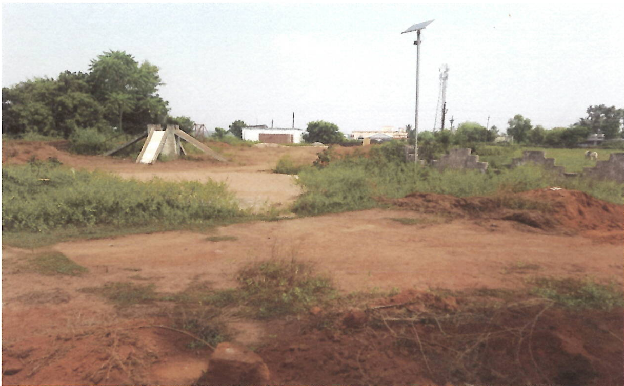
Const. Of Children Park at Narangarh (Work on progress )
