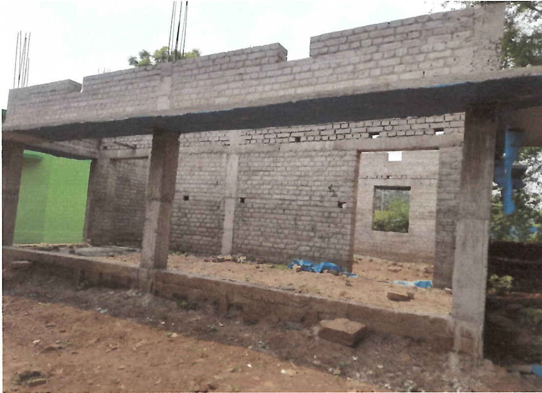
Const.of Additional class room at Narangarh UP School (Work on progress)
