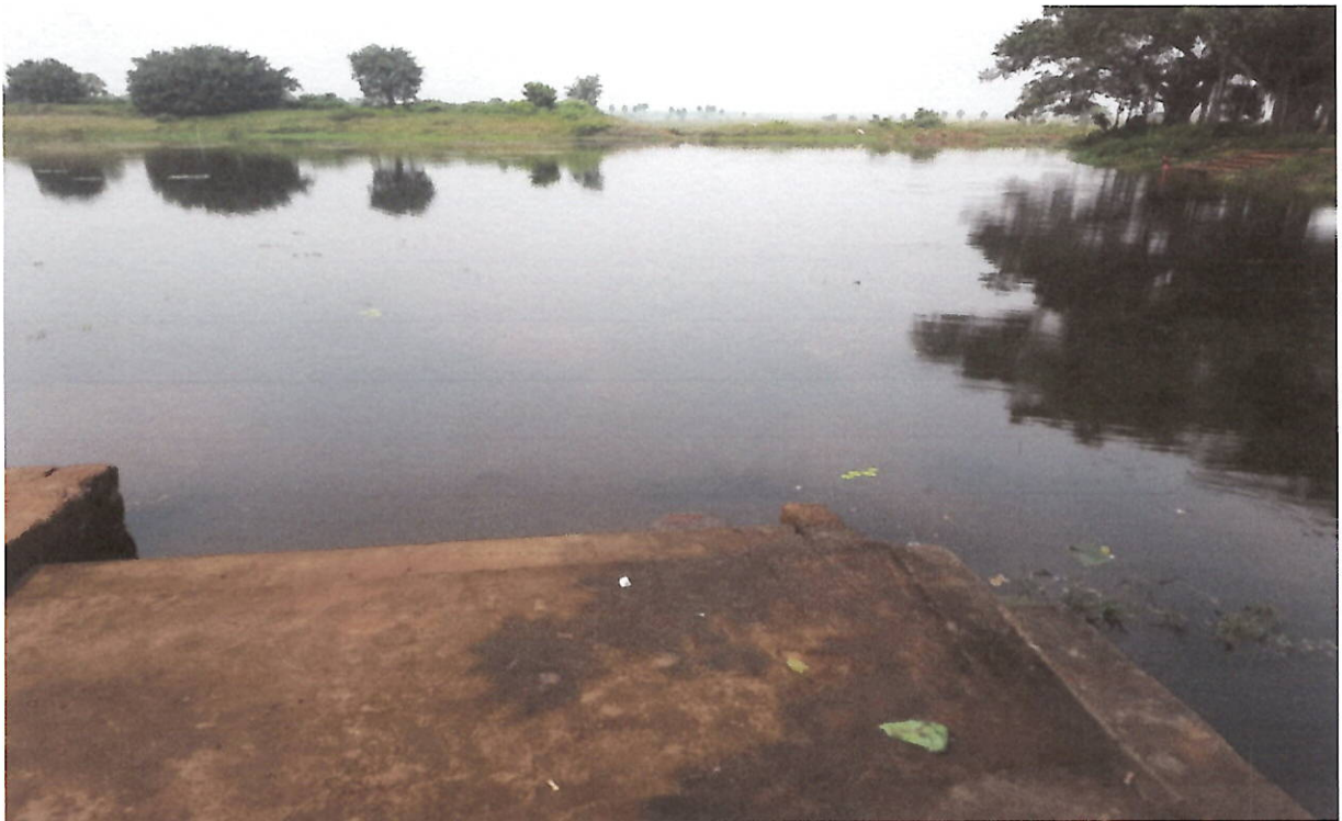
Renovation of Gajabaran Pokhari, Narangarh (Completed)
