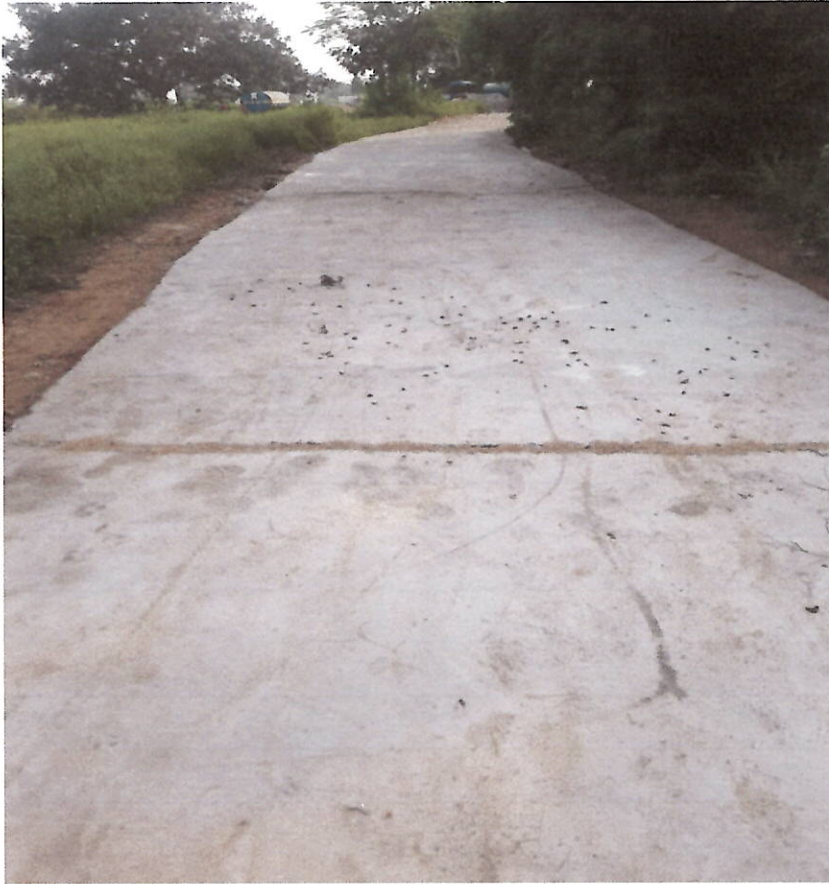
Repairing of CC road from Tapanga Railway station to Kanchila (Completed )
