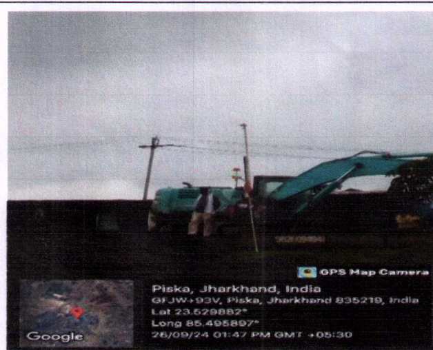
Photo 10: Fixed type sprinkling system installed at M/s Bansidhar Construction Private Limited Stone Crusher unit in Piska, Ormanjhi
