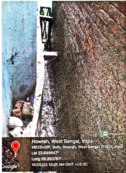
Bally Nursing Home out fall
