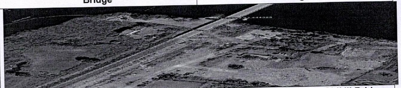
Fig. 5. Google Earth image showing sand stock on the right side of the Chikhili Bridge
