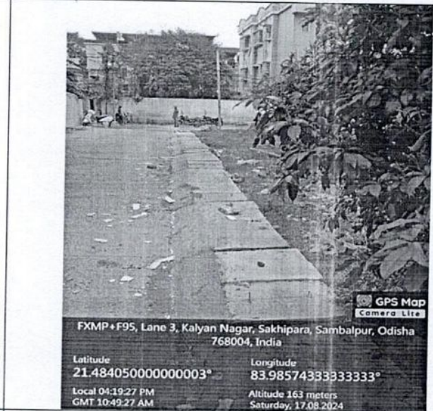
Fig. 2. Picture showing the vicinity of the drain to the boundary of Smt. Haripriya Patel
