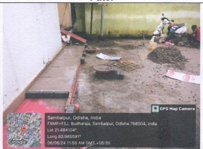
Fig. 4. Concrete slabs being casted to cover the open drains
