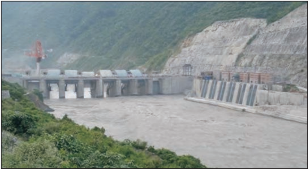
Figure 2.8: Hydel power project in Srinagar, Uttarakhand 44 .
