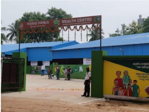
Figure 7: Entrance with concrete flooring and slope
