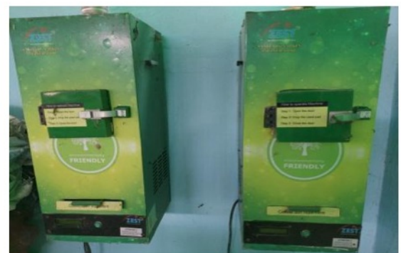
Figure 34: Incinerator at MRF
