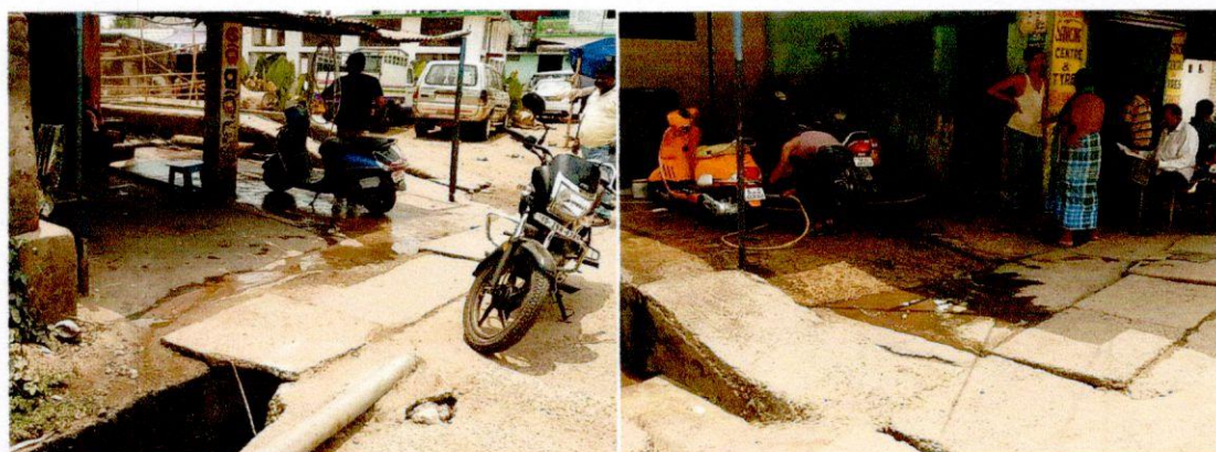
Views of operating vehicle washing stations discharging wastewater into municipal drain at Naya Idgah
