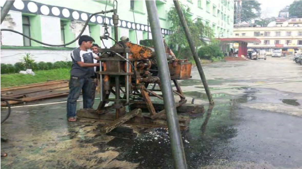
Drilling on Progress at Tashiling Secretariat
