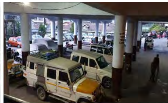
G-2 floor of existing MLCP
