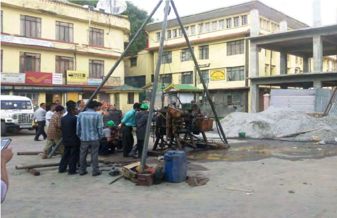
Drilling on progress
