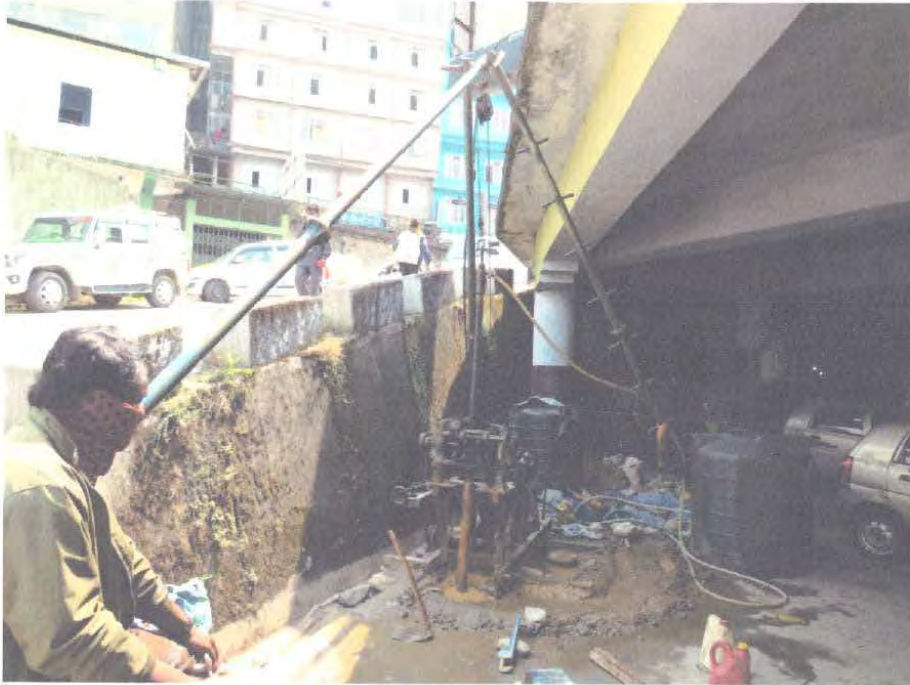
PHOTO;- DRILLING UNDER PROGRESS AT LOCATION BH-05.
