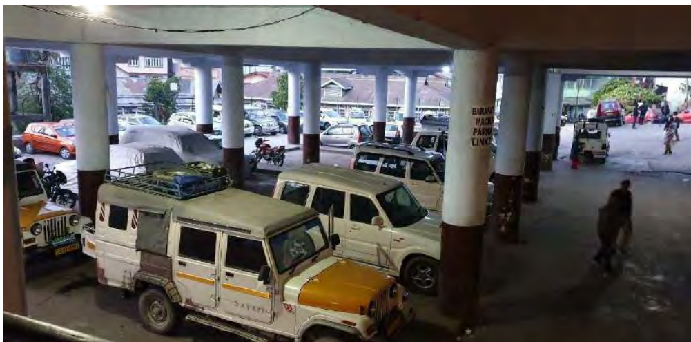
Figure 5: Existing MLCP, at Old West Point School Area
