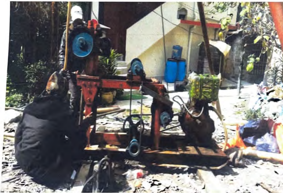
Photos:- Diamond core drilling of Borehole number 02 behind Old West Point School building at Gangtok, East Sikkim
