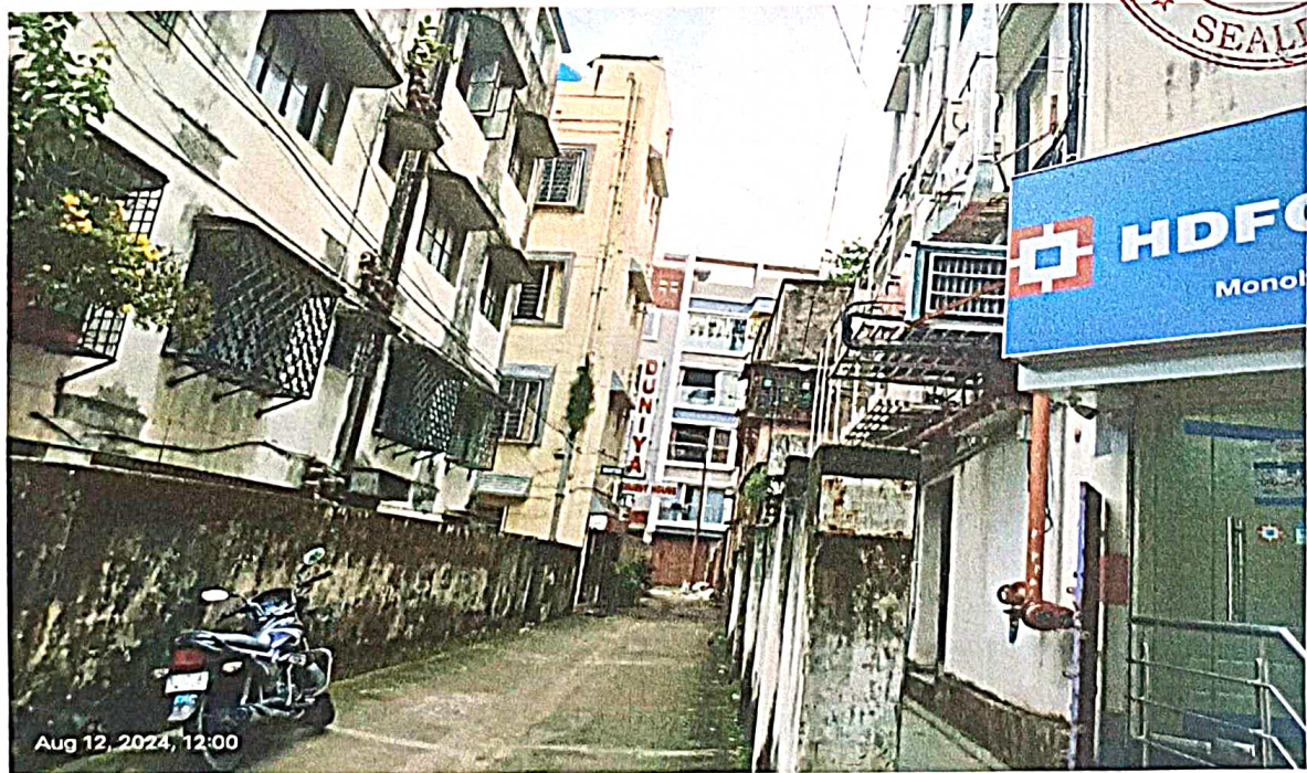
View of gap between the Bank & the complainant's residence.
