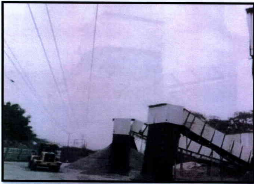
Figure-2(a): Chute from top of discharge point
