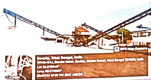
Pic. 3 Uncovered machineries of the unit
