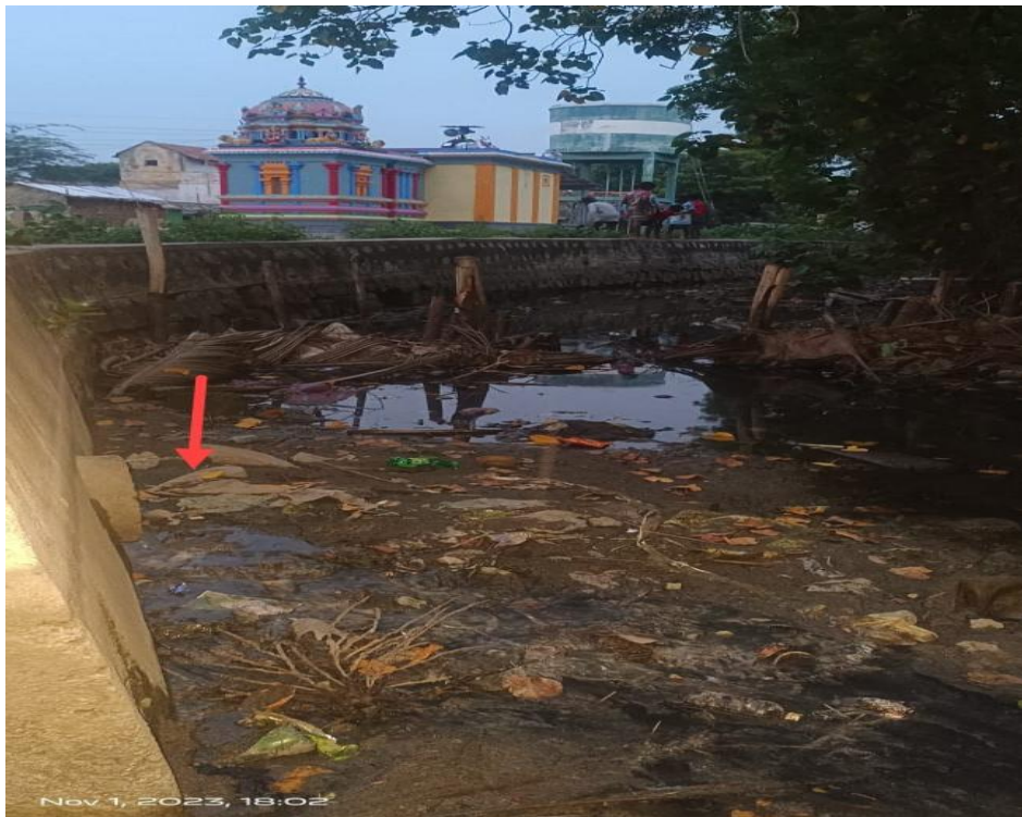
Bathroom sewage discharged into agriculture canal
