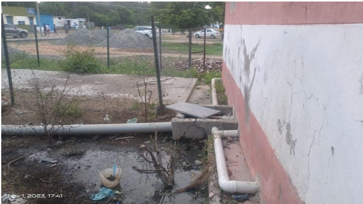
92m pipeline through which bathroom sewage discharged
