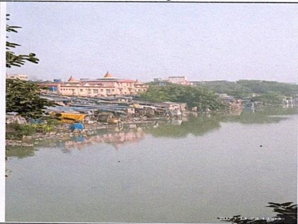
Shanties constructed encroaching the banks of the canal
