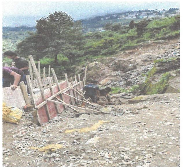
Under construction road from Mukti Dham towards Dumping ground
