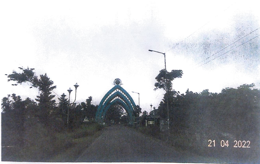
Photo 9: Digha Gate on NH-116B
