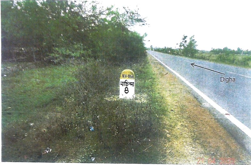
Photo 8: NH-116B towards Digha
