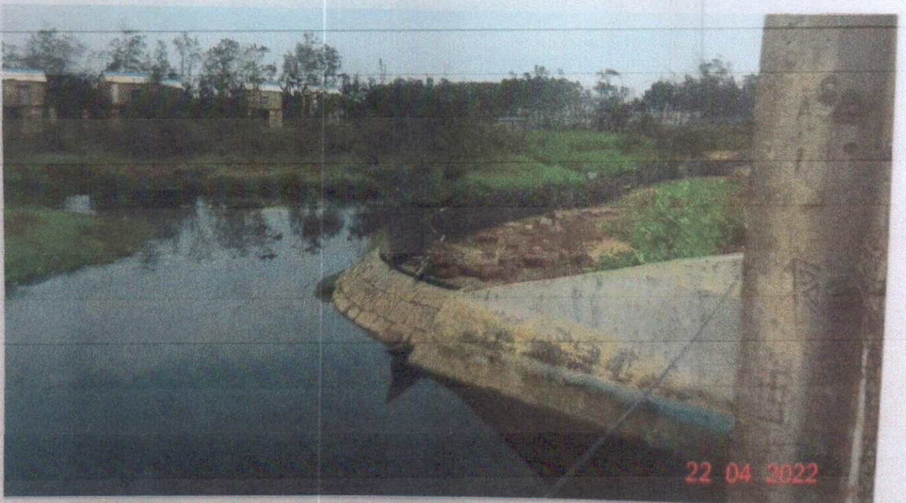
Photo 23: Present view of Jatra Nala.
