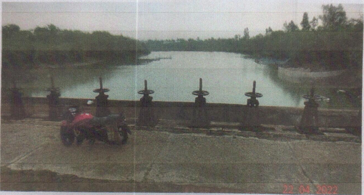
Photo 29: Sluice restricts tide flow near Sankarpur
