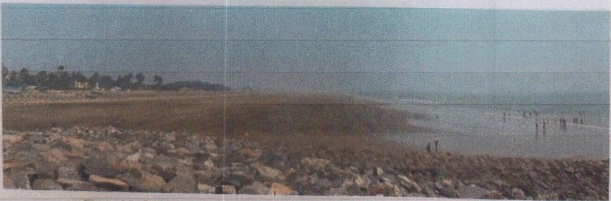
Photo 30: Structural measures to arrest erosion in the beachface, Digha east.
