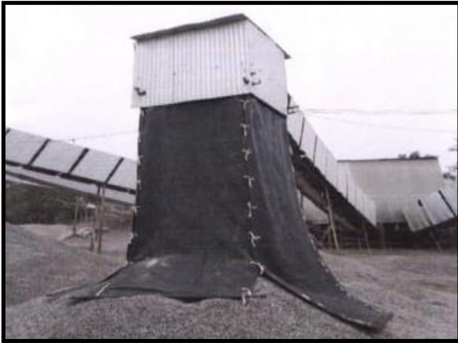
Figure-2: Chute from top of discharge point
