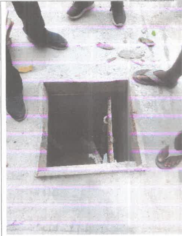
Waste water collection sump in the drainage line
