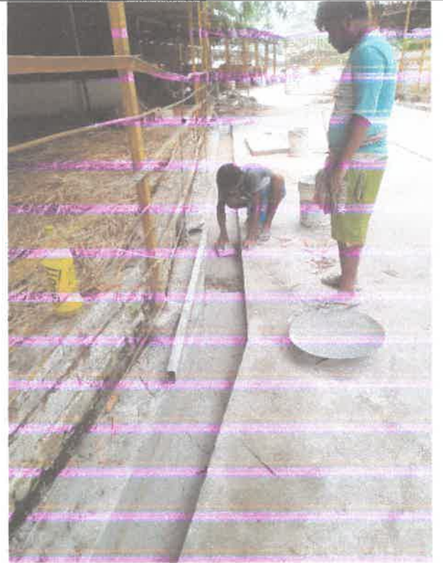
Construction/renovation work of internal drainage system is under progress
