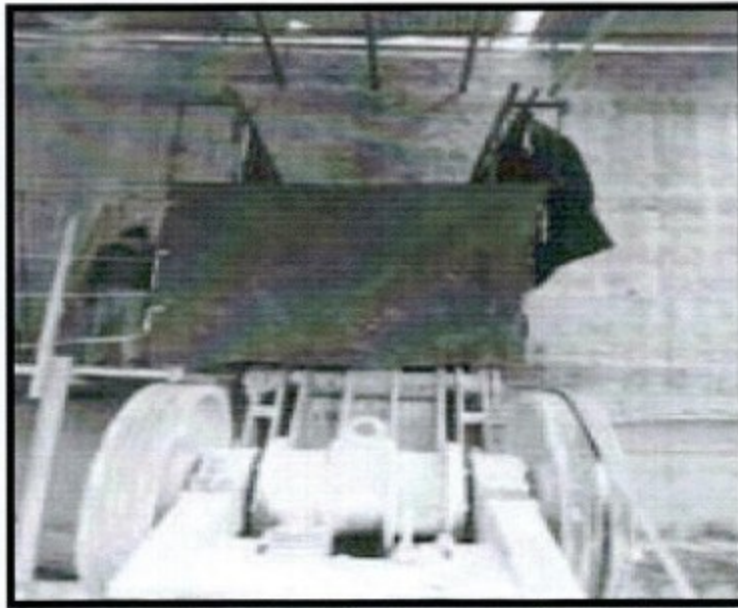
Figure-1: Covering of Primary/Jaw crusher
