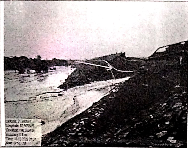
Breach site of Ash Pond-C
