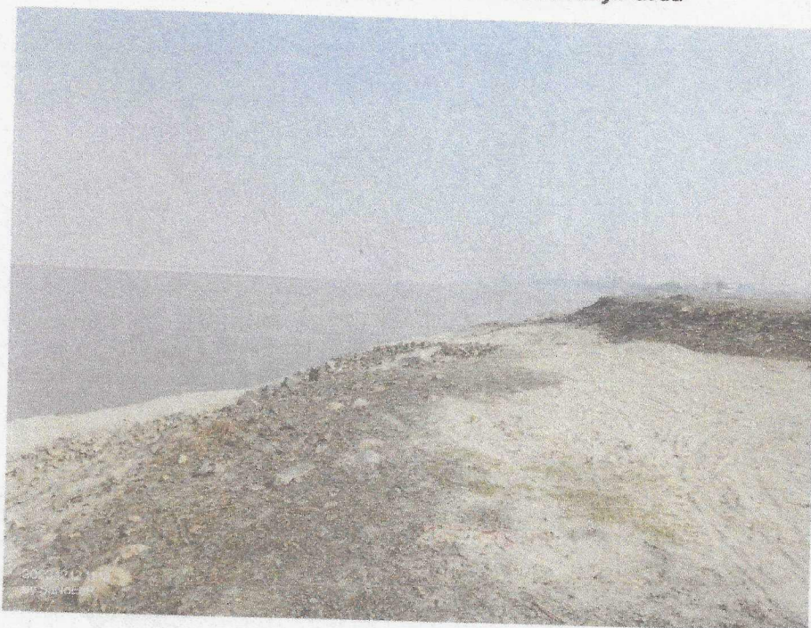
Photo 2: - Boulder Storage Area at Chhota Toufir
