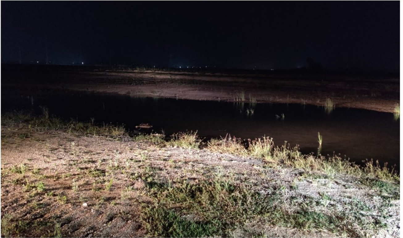
Ongoing works for Reservoir at Yedula Village
