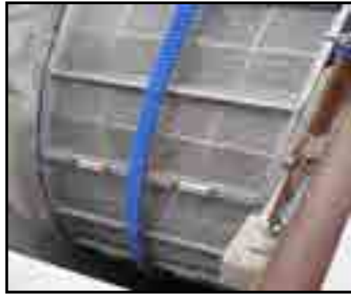
Figure 5-154: Fine Intake Screen
