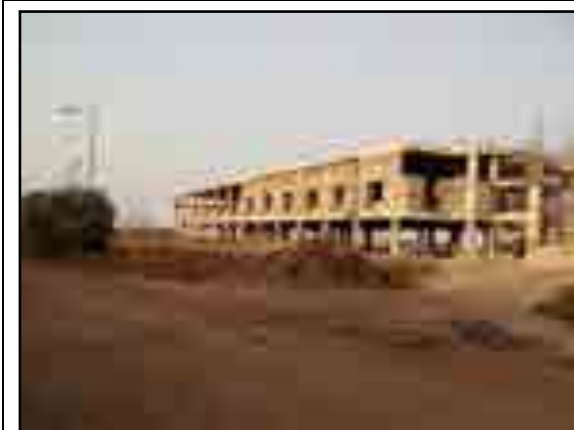
Exhibit 2-14: New MCC Building
