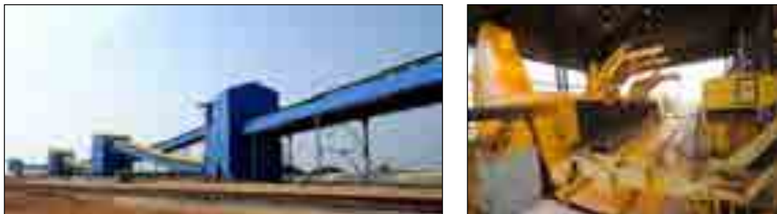
Exhibit 2-3: Covered Conveyor Belt and Wagon Tippler
