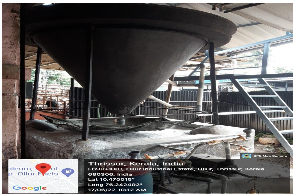
Figure 5 - Hopper bottom settling tank and sludge drying bed
