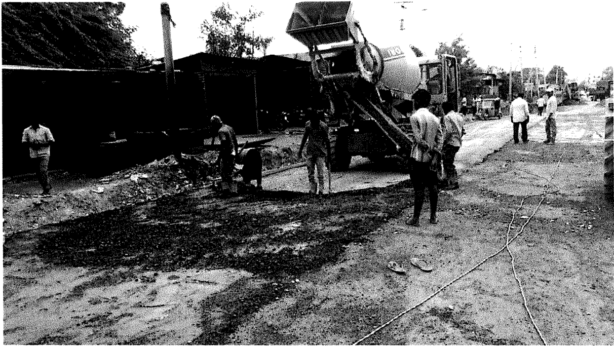
PHOTOGRAPH SHOWING THE STARTING OF ROAD WORK
