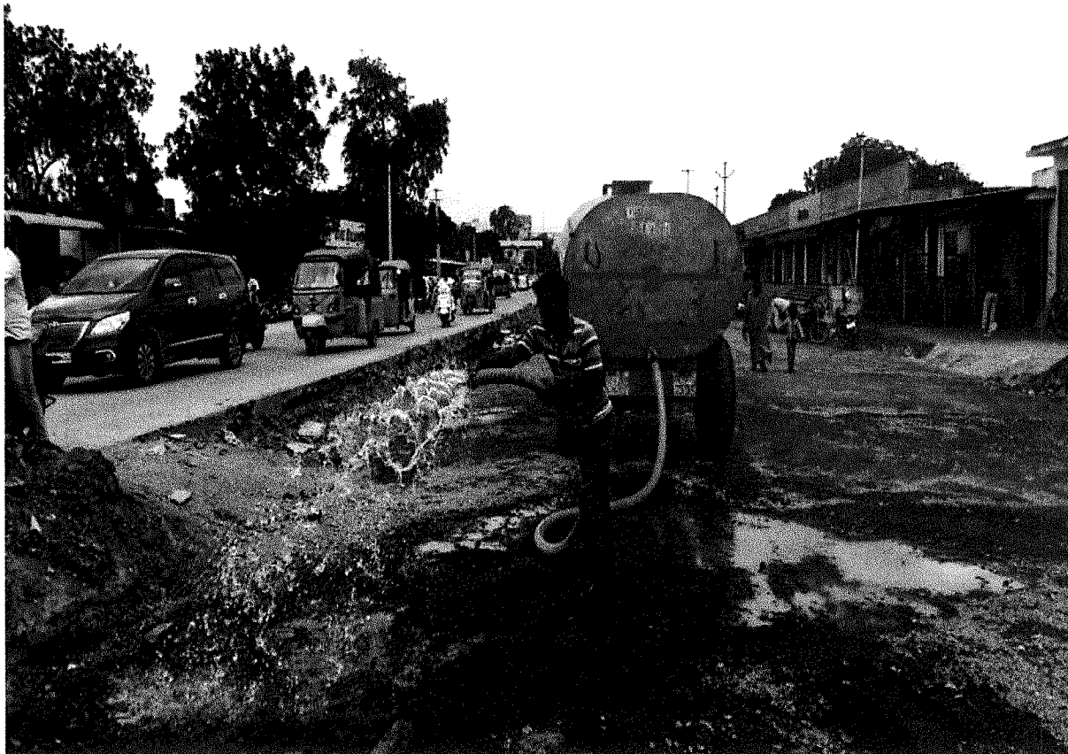
ADDITIONAL WATER TANKER PROVIDED BY THE R&D DEPARTMENT TO SUPPRESS THE DUST GENERATED DURING THE ROAD CONSTRUCTION ACTIVITY
