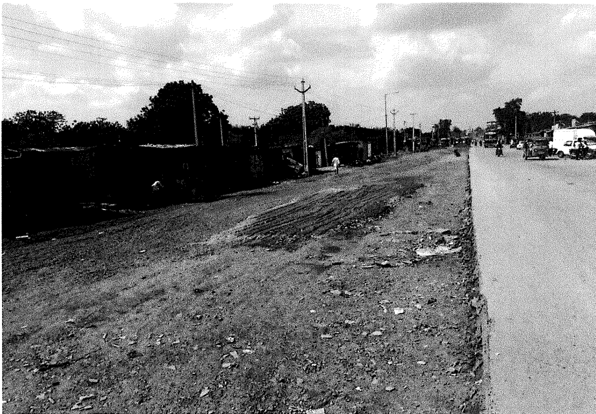
PHOTOGRAPH SHOWING THE COMMENCEMENT OF REMAINING ROAD WORK
