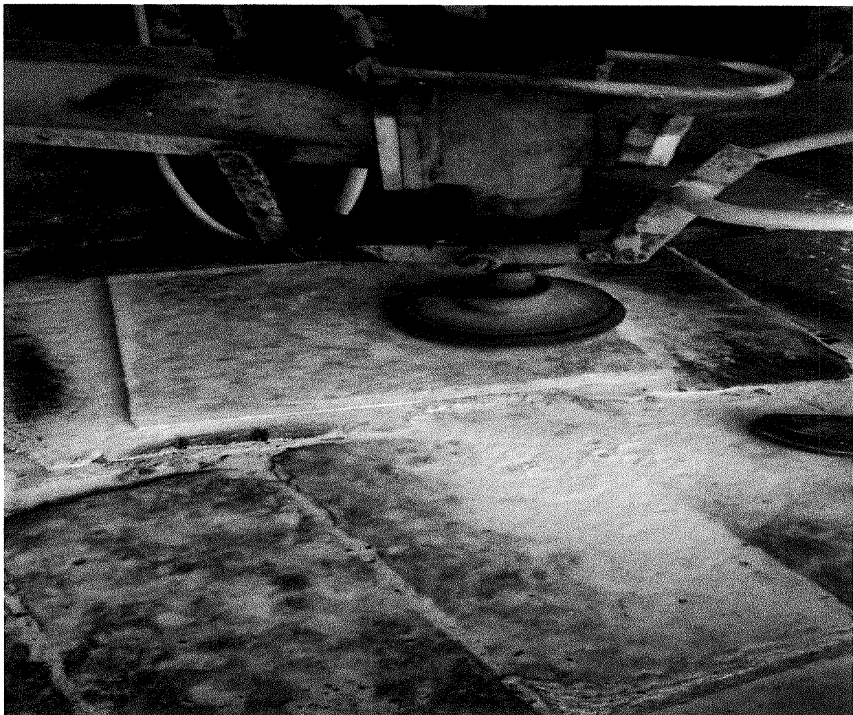
WATER SPRINKLING SYSTEM DURING STONE POLISHING OPERATION
