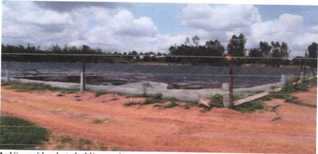
Photo 4 : View of leachate holding tank
