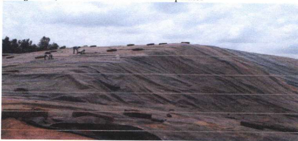
Photo 2: View of landfill of phase 1, covered with HDPE sheet
